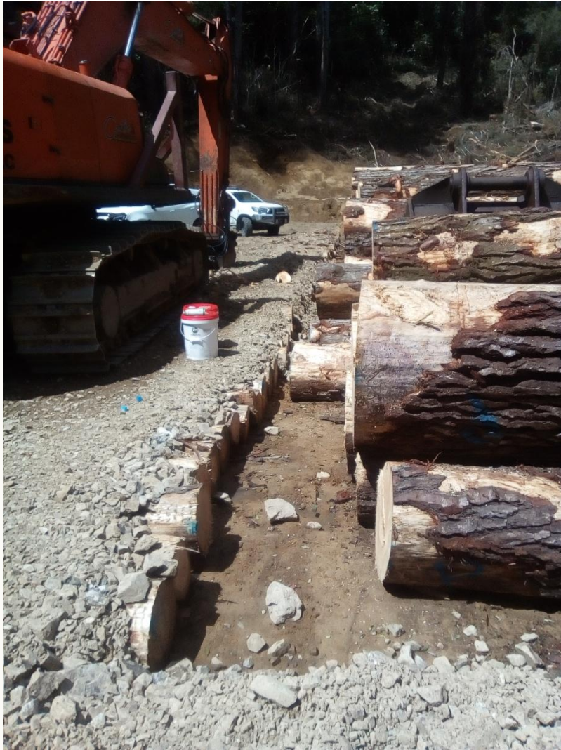
Corduroy skid site, logs laid with gravel to reduce dust and mud
