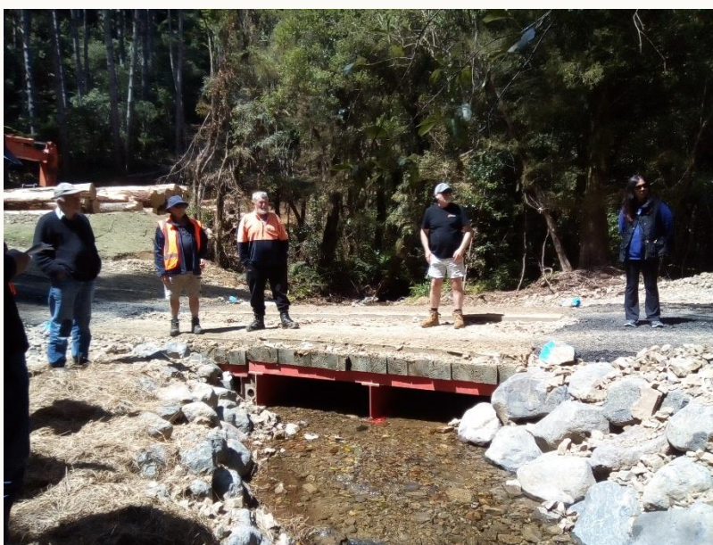
Temporary bridging that can be removed when the skid site is closed.
