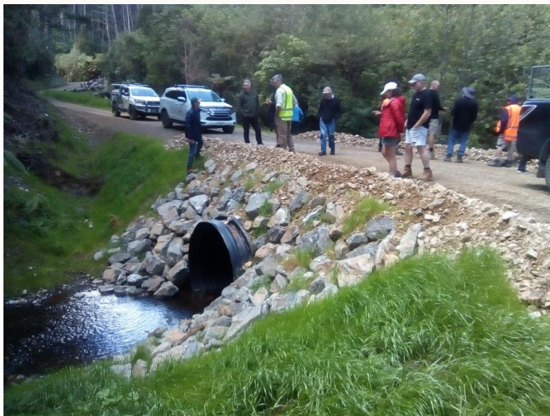
Reinforced culvert facing to stabilise the slope
