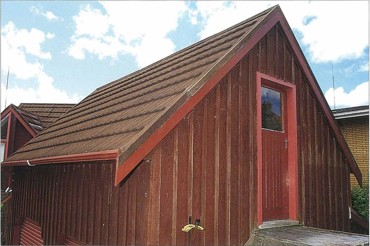
**Fig. 15 - Garage clad in New Zealand grown *Cryptomeria*, Rotorua.**
