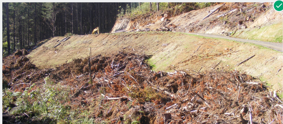
A slash bund intercepts sediment before it reaches the river.
