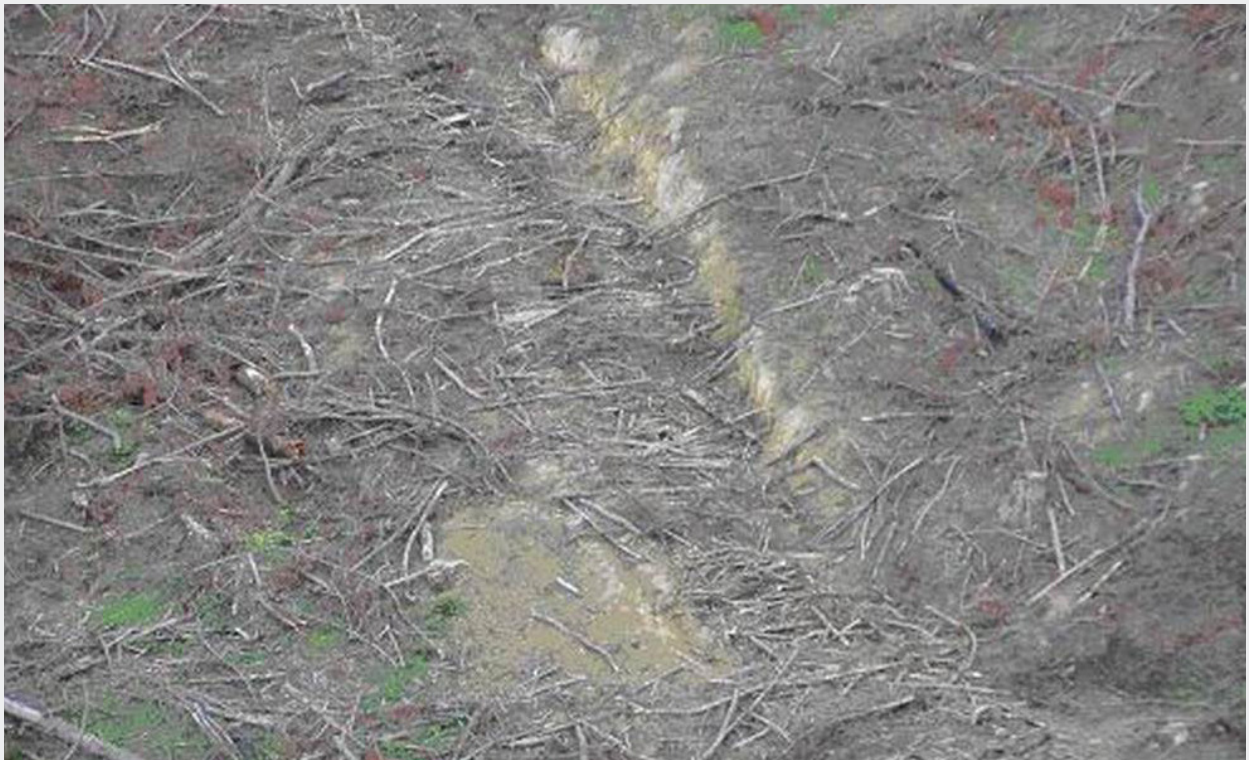
Slash cover on track to minimise sediment movement.
