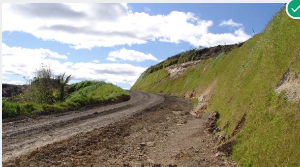
Good example of hydro-seeding on a steep roadside.
