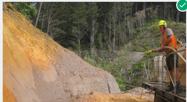
Cut batter being hydro-seeded to assist stabilisation .
