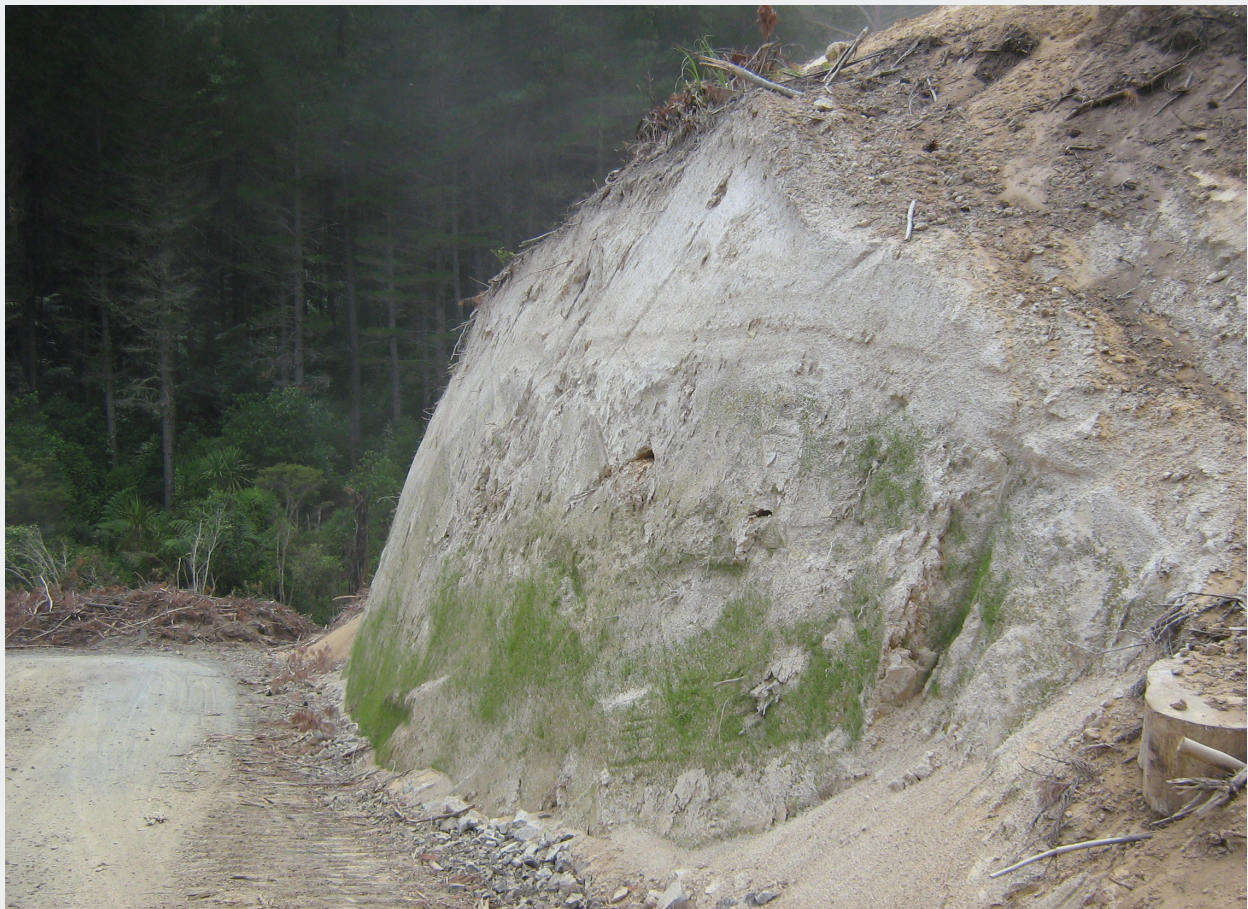
Success of hydro-seeding is dependent on weather and soil moisture conditions. Hydro-seed has germinated only on the lower section of this cut batter where soil moisture was highest.
