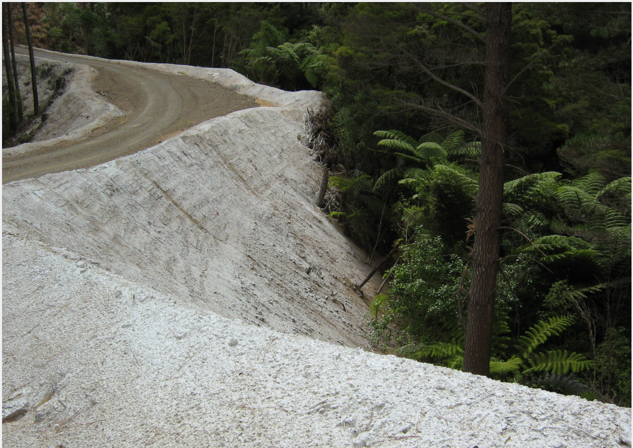
A recently hydro-seeded fill slope.
