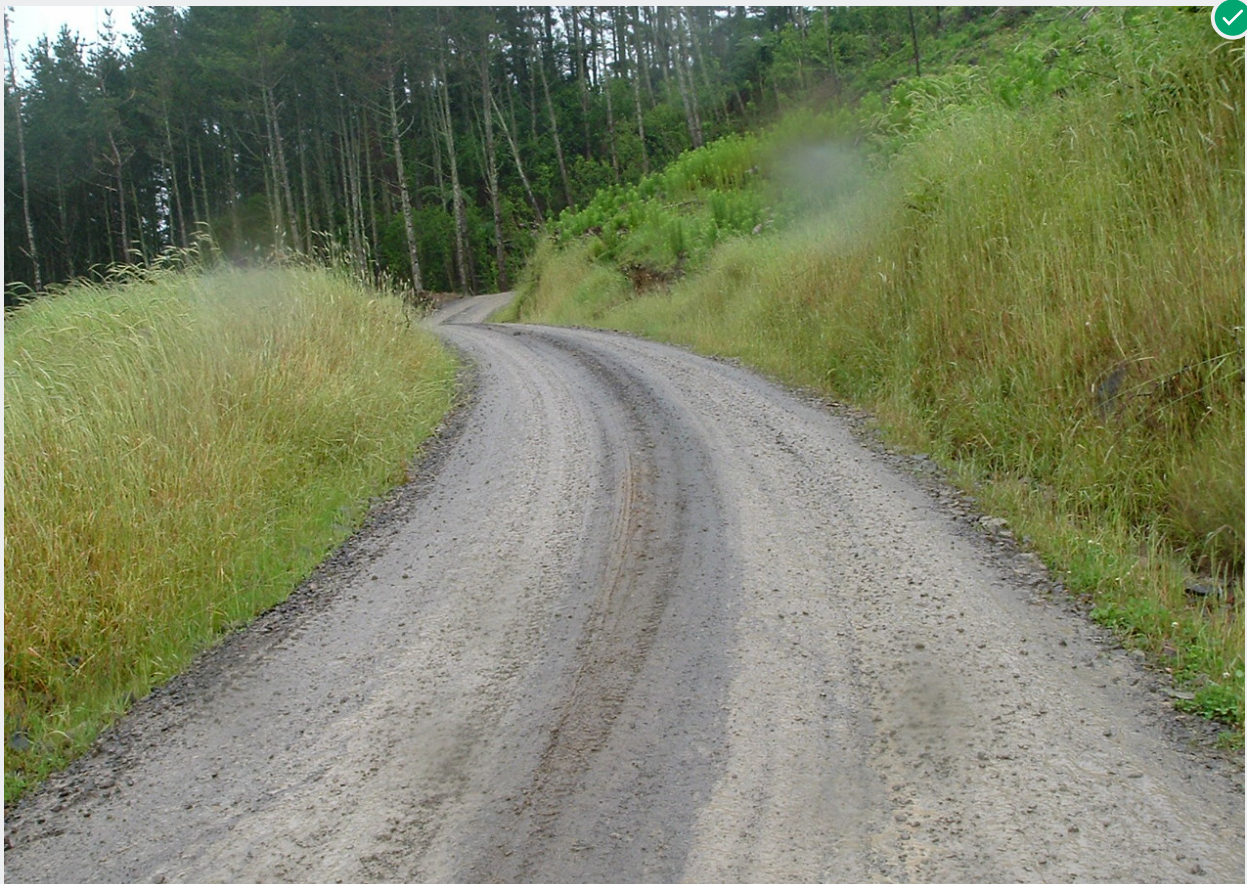
A good example of grassing to protect road edges from raindrop impact.
