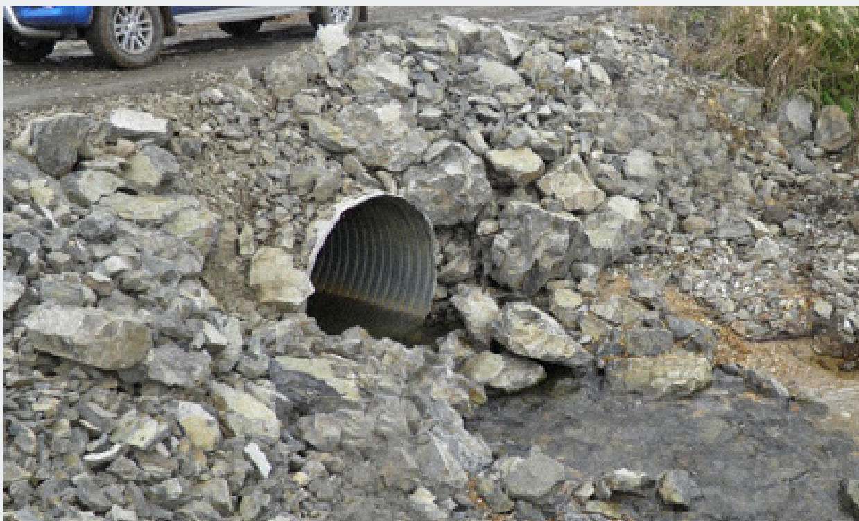
Culvert installation.
