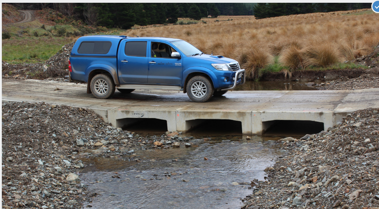
A well-constructed drift deck.
