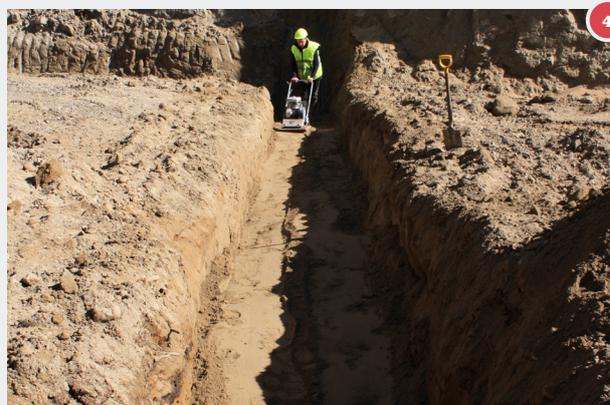
Compacting fill around and over the culvert.
