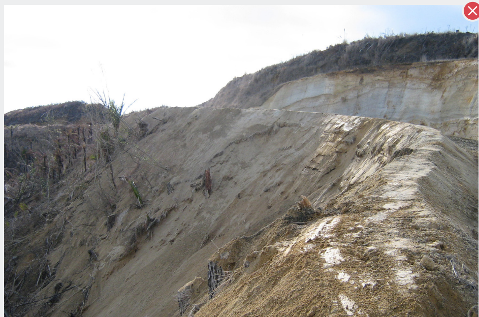
This berm is too large for the slope and road verge. Material is spilling from it.
