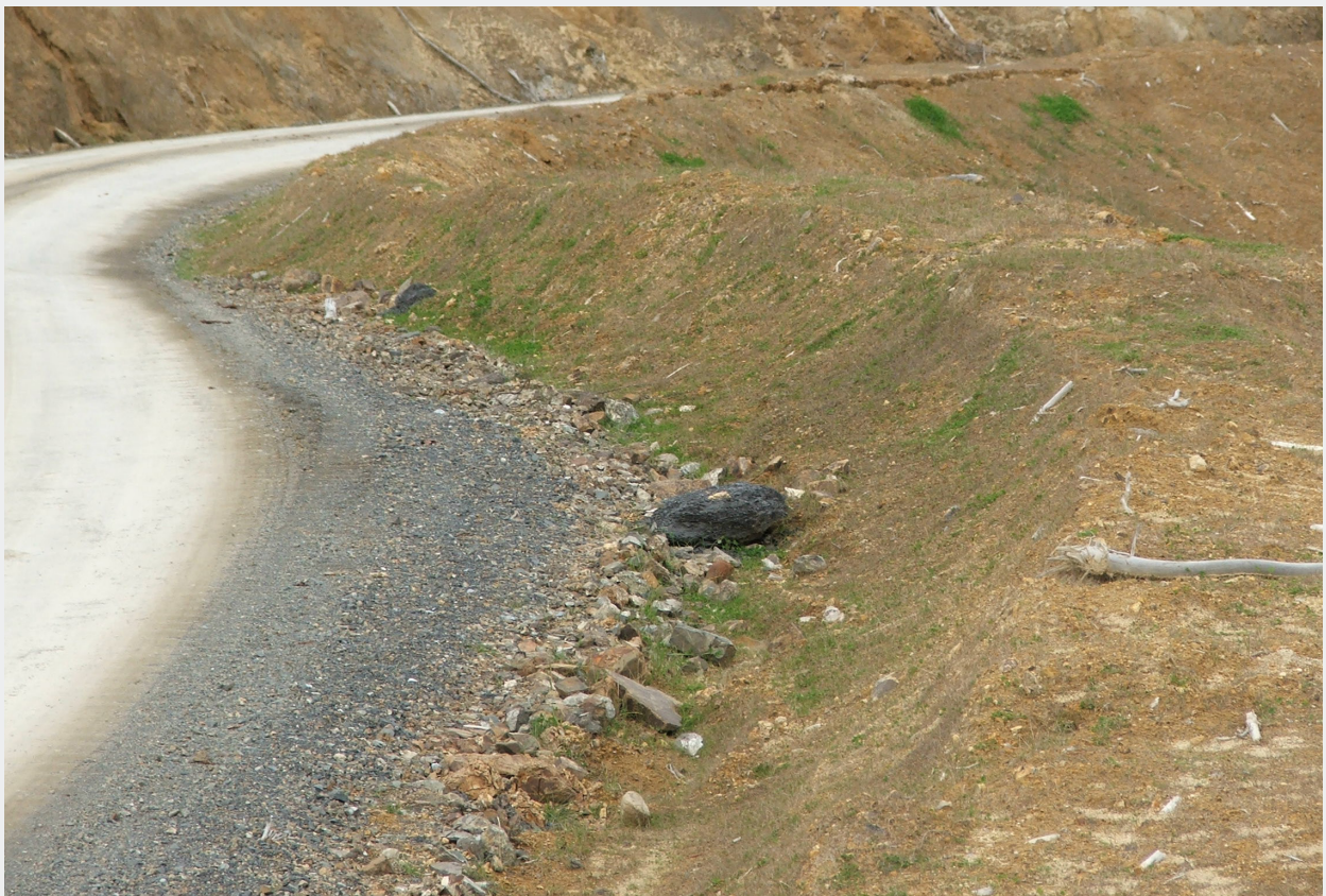
Low compacted berm.
