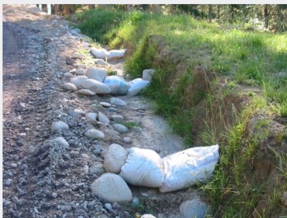
Water table check dams.
