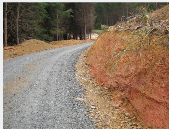
Water table with road base course used for rock armouring.
