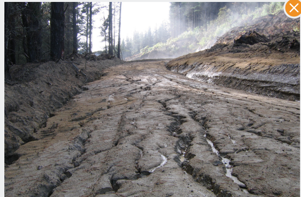
New earthworks formations need to be surfaced to prevent erosion.
