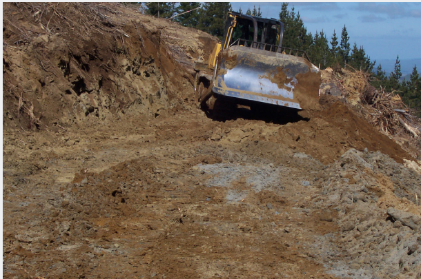
Dozer constructing a pilot roadway.
