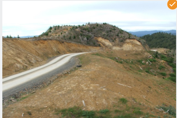
Example of well constructed road.
