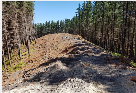
Road corridor after road-line salvage and prior to clearing and stripping.
