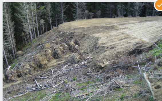
An example of good stump placement. Stumps have been placed on a shallow bench away from standing trees and the construction fill during clearing and stripping.
