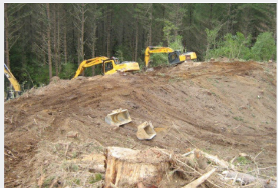
Excavators clearing vegetation and stripping topsoil ahead of landing construction.
