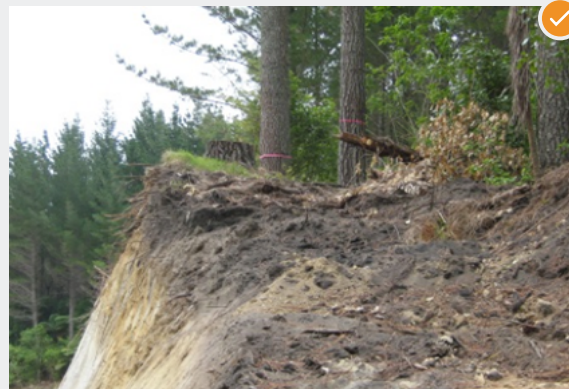
Example of good road-line salvage with a sufficient number of trees removed providing adequate width road formation.
