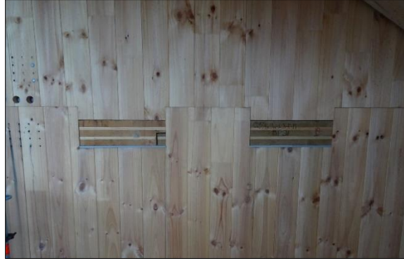
Figure 2: Castellated connection in NZ CLT Building (c/o Sam Leslie)
