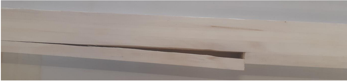
Photograph 2: Failure starting with Finger-joint failure on tension edge, Beam 289946
