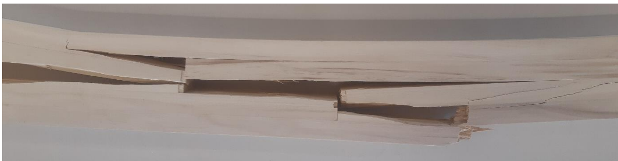
Photograph 1: Typical failure starting with Finger-joint failure on tension edge then progressing through the inner finger-joints, Beam 289947.
