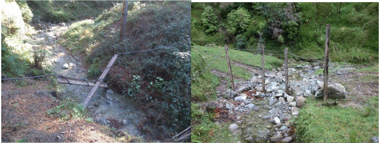
Figure 22: Left - Gisborne slash trap in a headwater stream using crossed railway irons embedded in the stream bed. Wire rope is wrapped around the railway irons and secured to radiata pine trees. Right - slash trap installed using vertical railway irons. Wire rope is threaded through the irons and secured either to mature trees or with deadmen (buried anchors).
