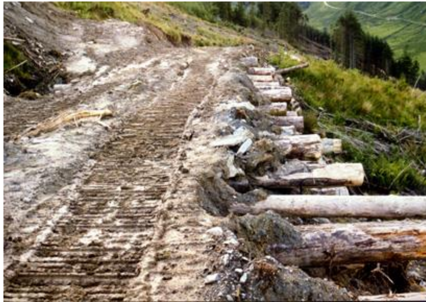
Figure 14: Corduroy road, where logs are used to help support road construction on soft or unstable slopes.
