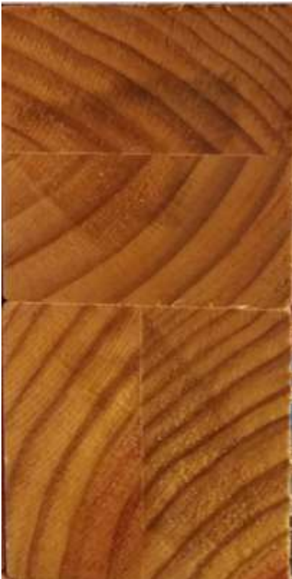
4b: Cross-section appearance using spot-test for zinc tracer chemical showing incomplete penetration of sapwood. This is a fail.
