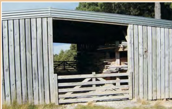
Purpose-built shed for air-drying sawn black beech timber.
