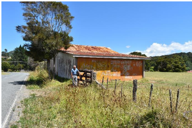
Figure: 19 - John McGee stands by a 'lean-to' addition to a shed on Robert Hayes' property on Omaunu Road in Kaeo. In 1968 John and the (late) former owner, Jim Leslie, cut and delivered two tōtara trees for use as beams in the lean-to construction.
