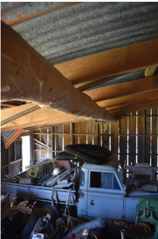
Figures: 22 & 23 – View to the large (butt) end of the 8.57m long tōtara beam, which rests on a piece of framing timber with house borer exit holes. However, no borer or rot is evident in any part of the untreated tōtara beam (N.B. the smooth natural round surface of the timber under the bark).
