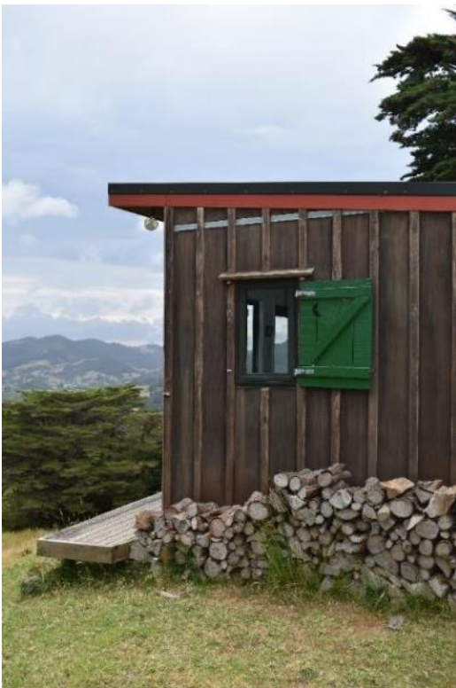
Figures: 16 & 17 – ‘Coloured’ pieces of totara timber (i.e. ones that are part sapwood/ part heartwood), were deliberately used in August 2009 as a performance trial of untreated tōtara in
