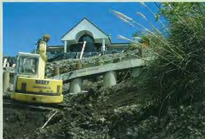
A reinforced concrete palisade wall is being constructed several metres inland of the cliff edge.
