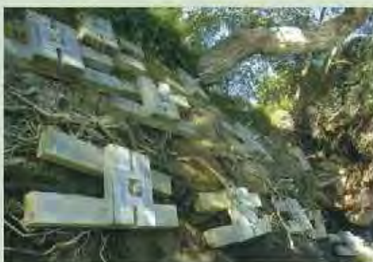
Engineering solutions to the problem of eroding cliffs in Auckland do little to enhance the natural character of the coastline.
