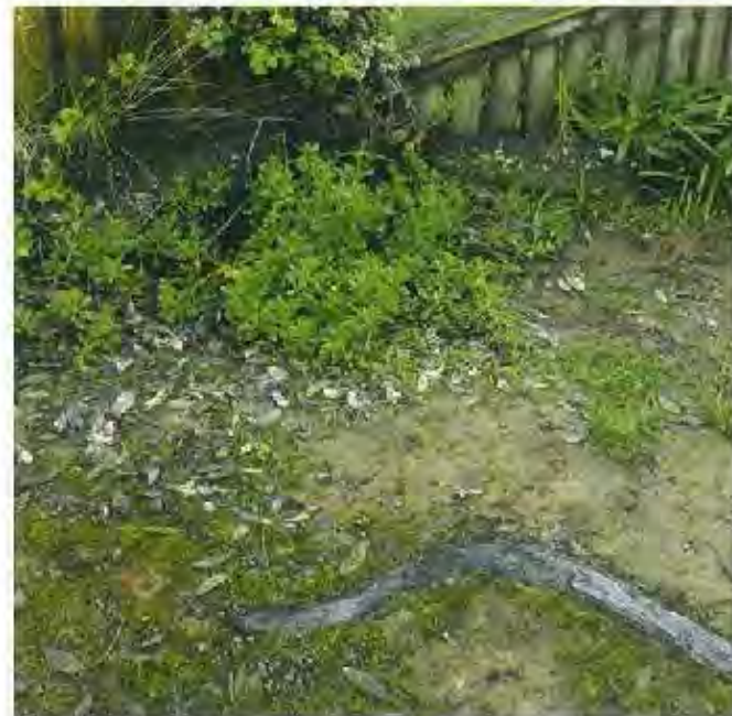
Top: Foundations and pavements in the vicinity of pohutukawa trees can be distorted by growing roots. Remedial work often involves removal of the tree.
