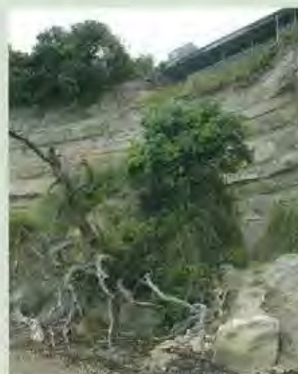
Debris at the base of a cliff with pohutukawa and other vegetation that has come down with a recent slip. The debris toe occupied by an interlocking mix of roots and branches is likely to be removed within months by high seas.
