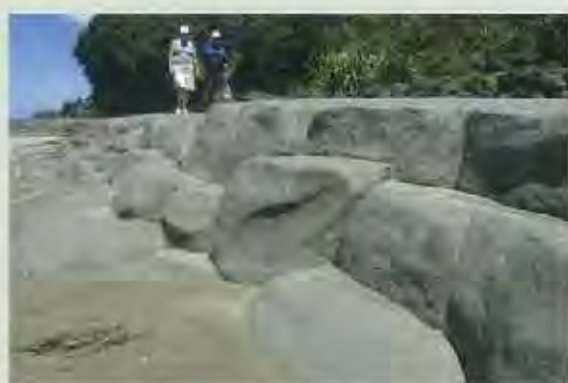
The sewer pipe running along the high tide line at Murrays Bay was covered with a layer of concrete to protect it from wave action. The structure is now acting like a low sea wall that could be reducing erosion at the base of the cliff. The concrete armouring of the sewer pipe was designed to look like the surrounding rock platforms and has become a popular walkway.
