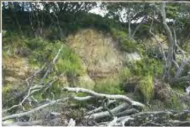
Pohutukawa-dominated bank undermined by high seas has collapsed on to the beach.
