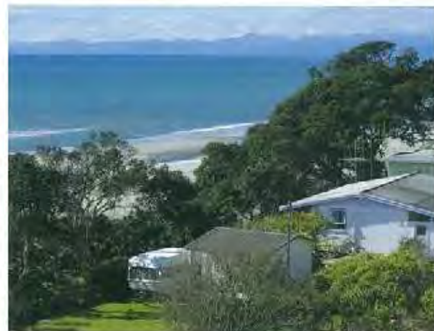
Houses are often built within a few metres of the edge of cliffs where only a single line of pohutukawa remain. In some instances, cracks in lawns open and close as trees are buffeted during high winds, indicating possible future failure.
